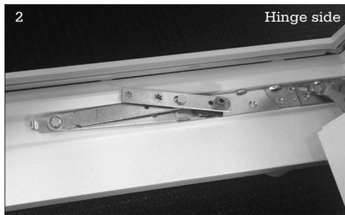
Open the sash sidehung. Click the frame and sash parts together and - at the hinge side of the cill - place the restrictor as show on the picture. When doing so, the retrofitting becomes straight forward.
