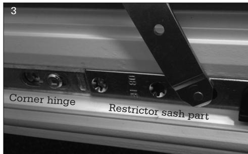
Underneath the sash, fix the sash part of the restrictor exactly next to the corner hinge hardware (3.5x25).
