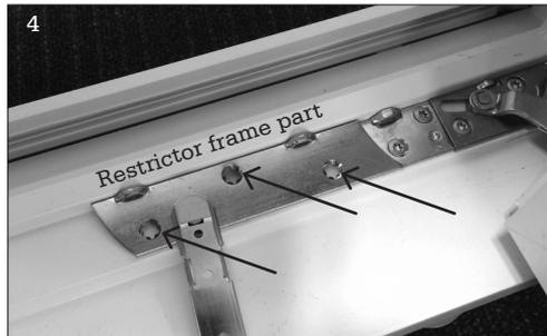
Fix the frame part of the restrictor at the cill as on shown the picture. Remember to pre-drill (3.5x25).
