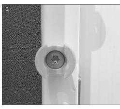
Mark out for placing of the window stay retainer 103mm below the centre of the frame-part - please see drawing.
